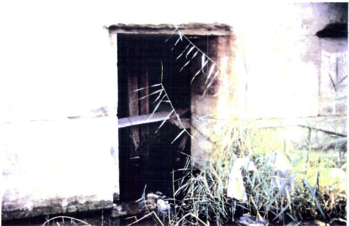
Plate 4: The entrance to the Sarcophagus Room. Note the wooden scaffolding supporting the interior of the room.
