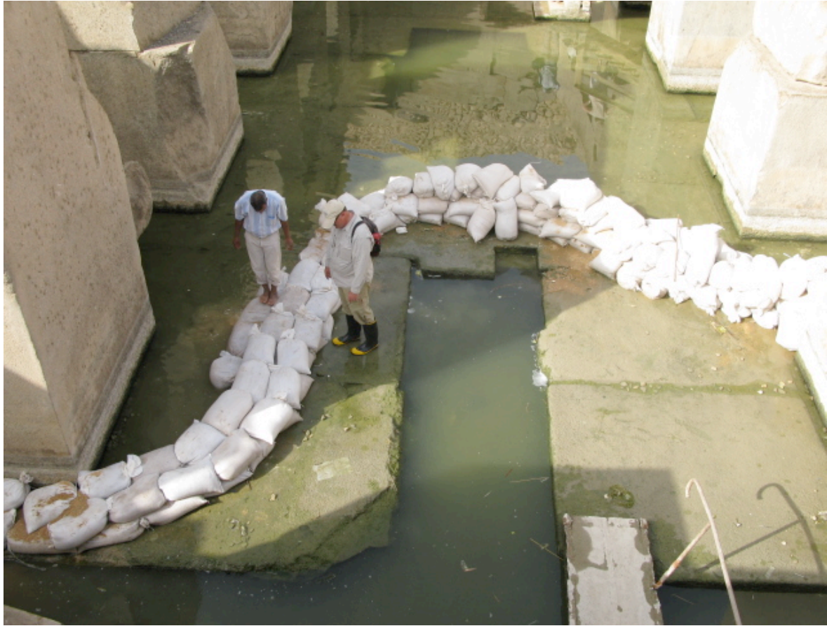
Sandbags surrounding western stairway of central island of the Osireion
