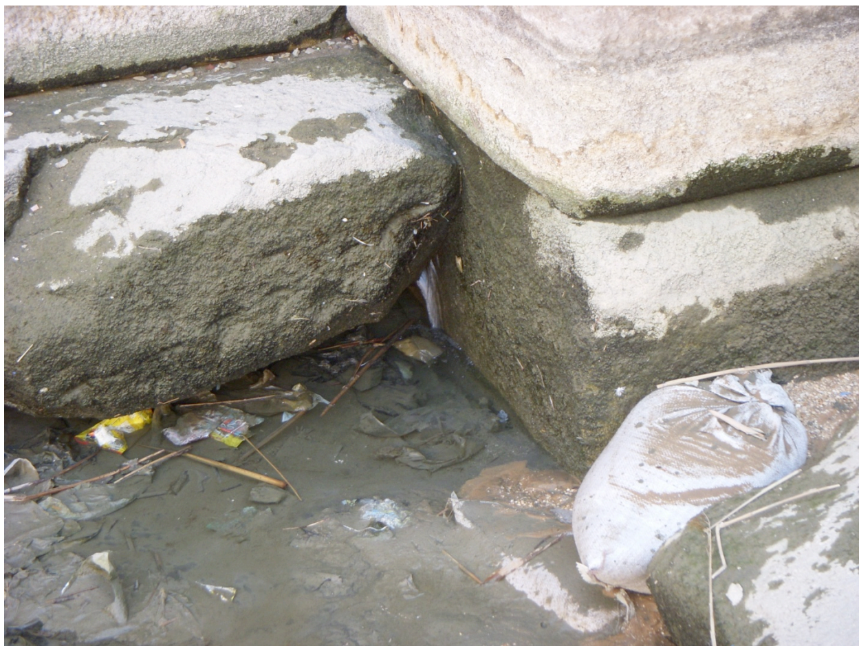
Rivulet of water flowing in by north pilaster on west wall of Osireion
