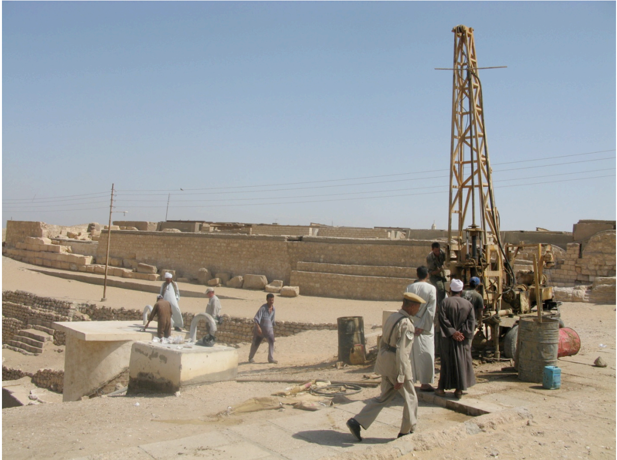
Drilling the Westerman Well
